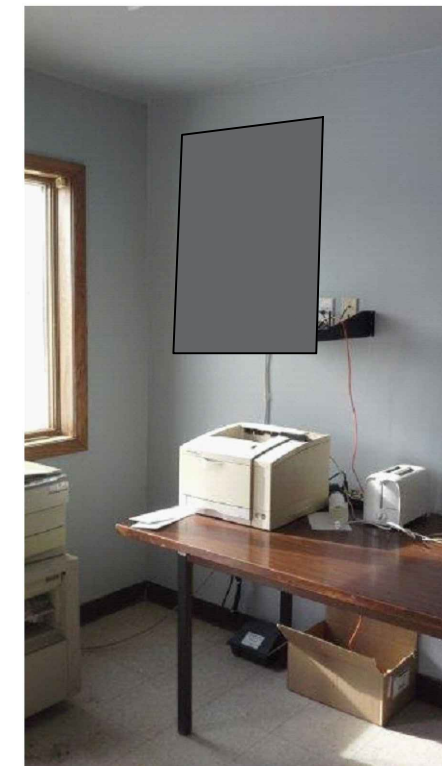
EXISTING RACK LOCATION
