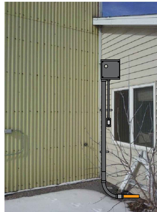
EXISTING BUILDING ENTRY BOX
