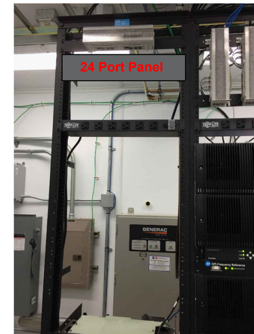
NEW PANEL INSTALLATION
